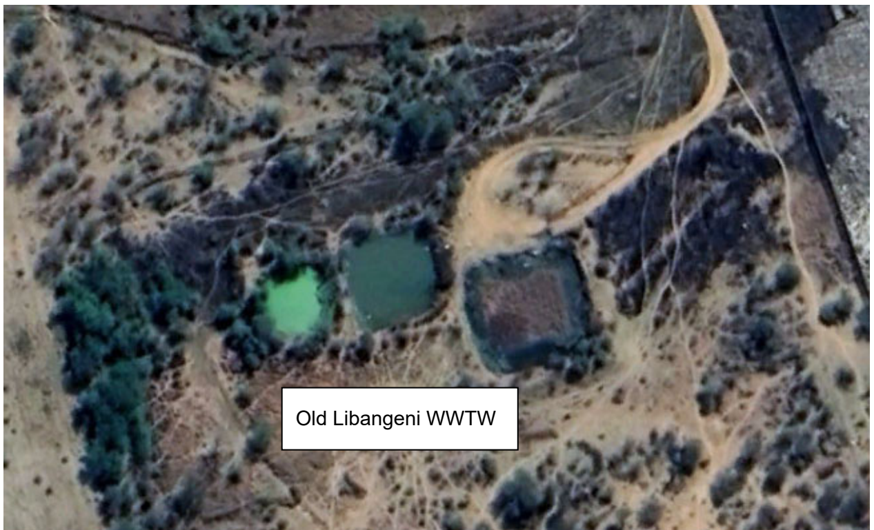
Figure 4.2: Old Libangeni 0.05Mℓ/day Retention Pond
